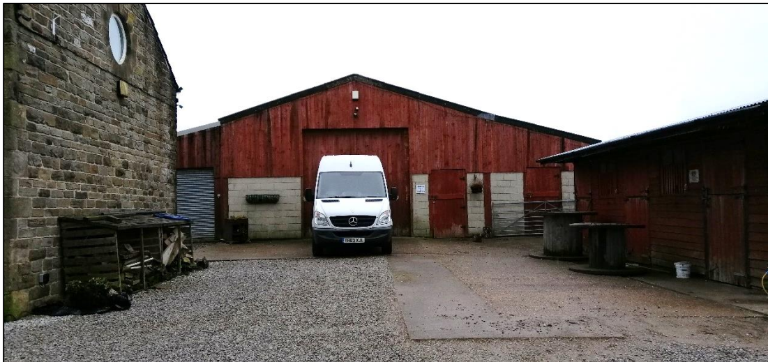
Plate 1. East elevation of barn showing hard surface in foreground
