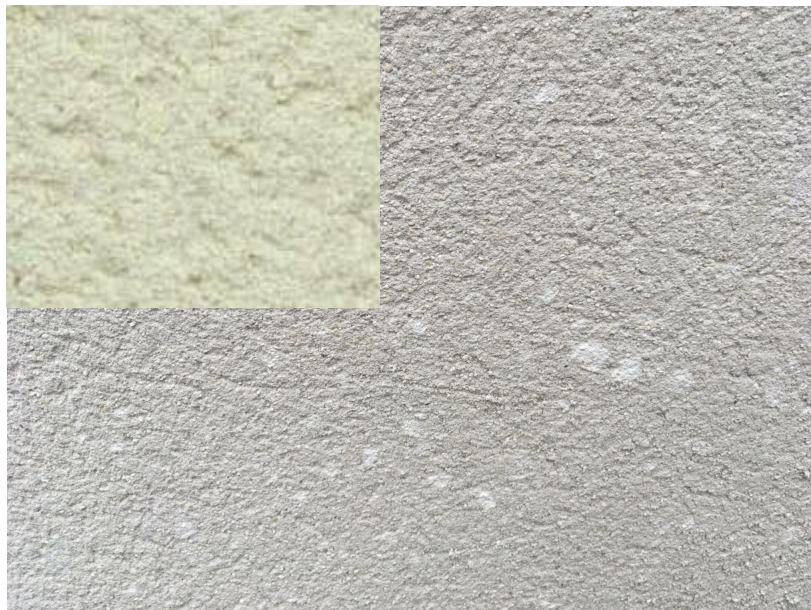
B. WALL 2 (inner gable)
