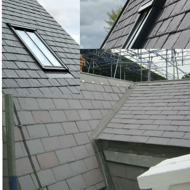
E. ROOF & ROOFLIGHTS
