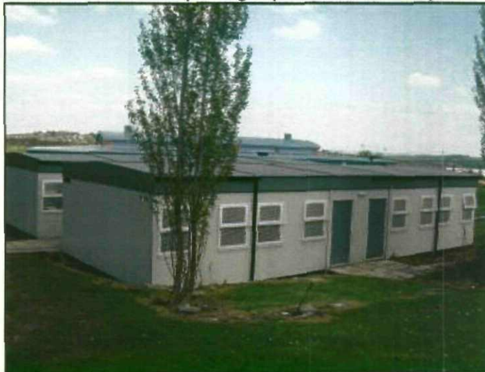
Plate 2 Two portokabin buildings
