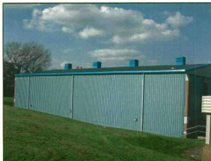
Plate 6 Barnsley College Honeywell – modern built structure to south western corner of building
