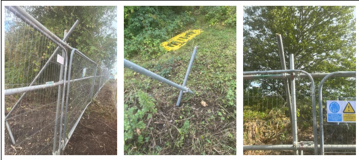
Figure A3.2: Examples of scaffold framework temporary tree protection barriers.
