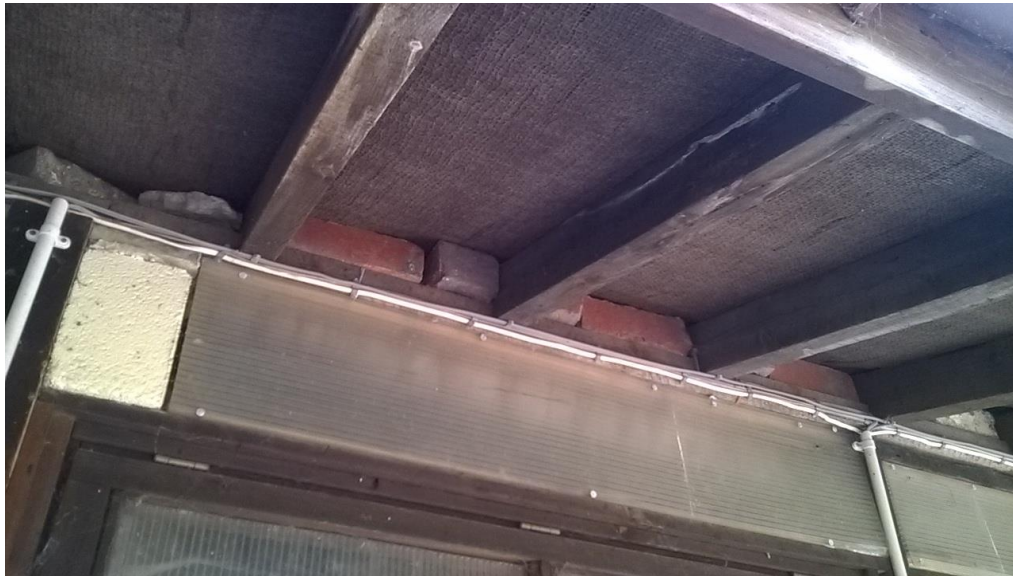
Plate 3 Bricks positioned to exclude swallows but bats can still access.
