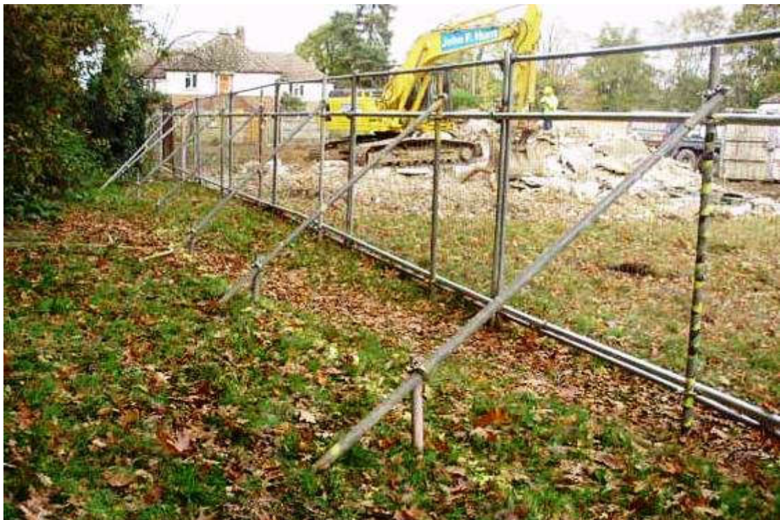
Figure 2: Photo of Fencing to BS 5837:2012
