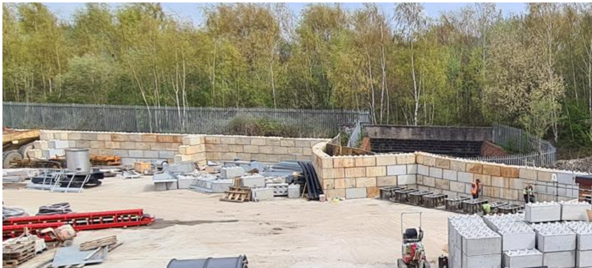
Figure 8. View of the site's eastern boundary
