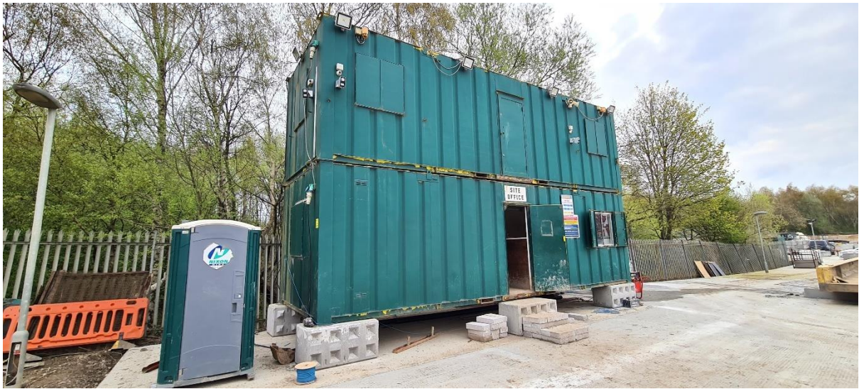
Figure 5. Photograph of the site office
