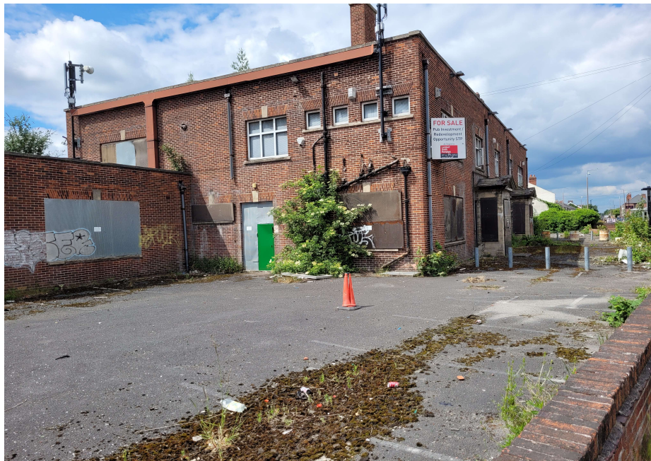
Area to east of hotel building
