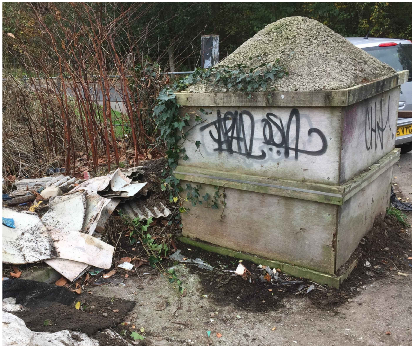
05 Existing Block and Japanese Knotweed
