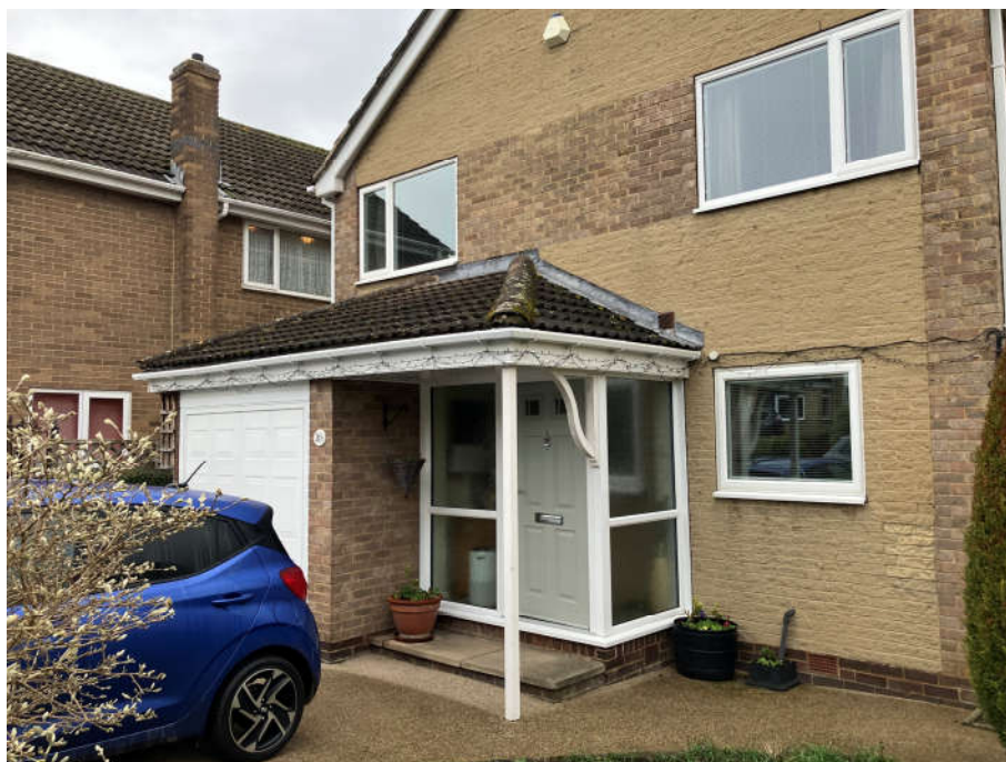
03. Detail of Front (South) Elevation.
