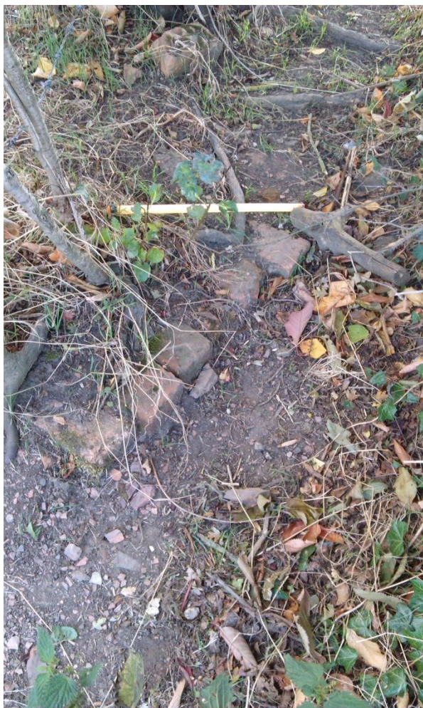
Plate 7 Un-frogged bricks within the kerbed trackway
