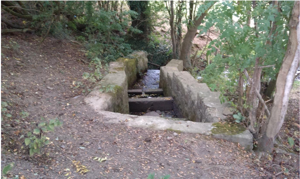
Plate 9 Drain outlet, looking Northwest
