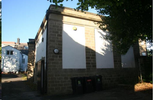
Existing Workshop/Store looking from Eastgate
