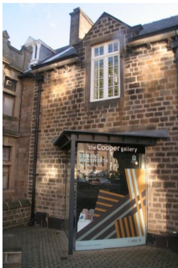
Modern glazed bays
