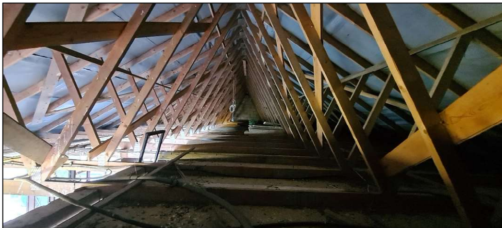
Plate 4. Roof truss construction
