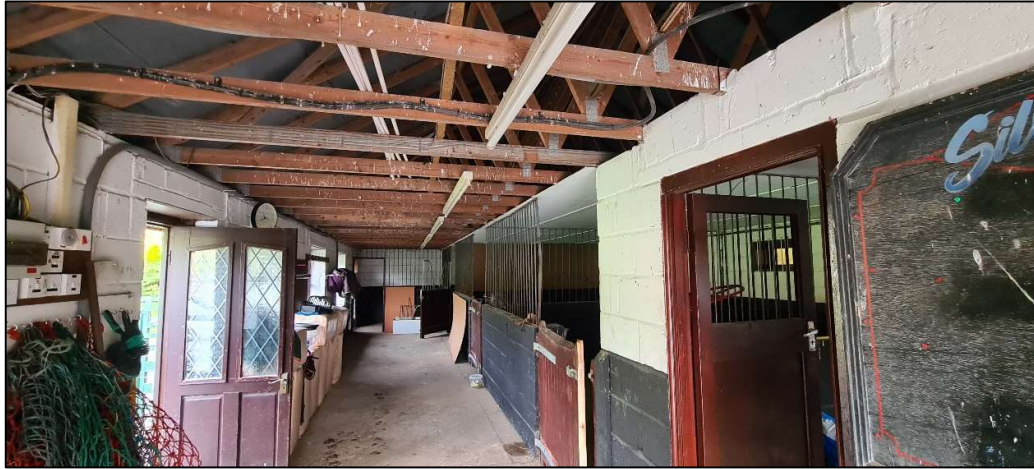
Plate 4. Roof truss construction
