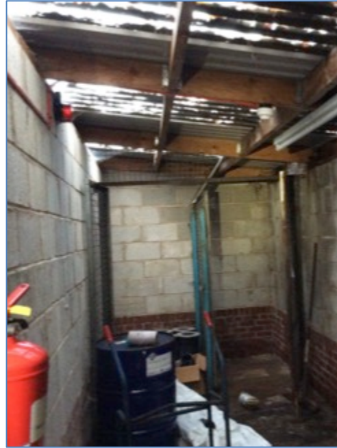
Photograph 29. Internal view of B27, showing corrugated roof panels
