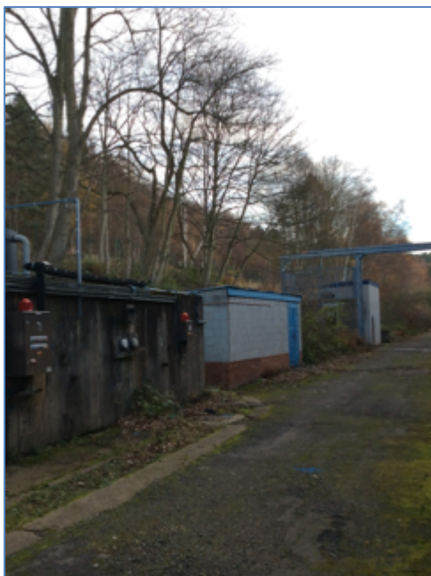
Photograph 11. Small buildings along a strip of woodland, with Wharncliffe Woods (TN7) in the background
