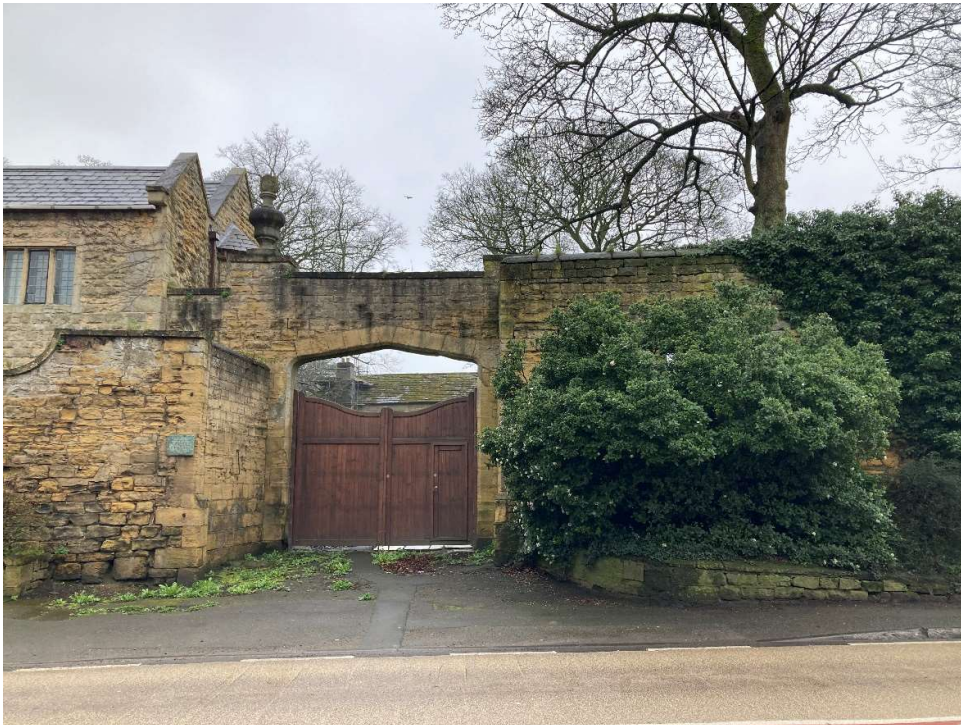
Plate 5 -Listed wall to the right
