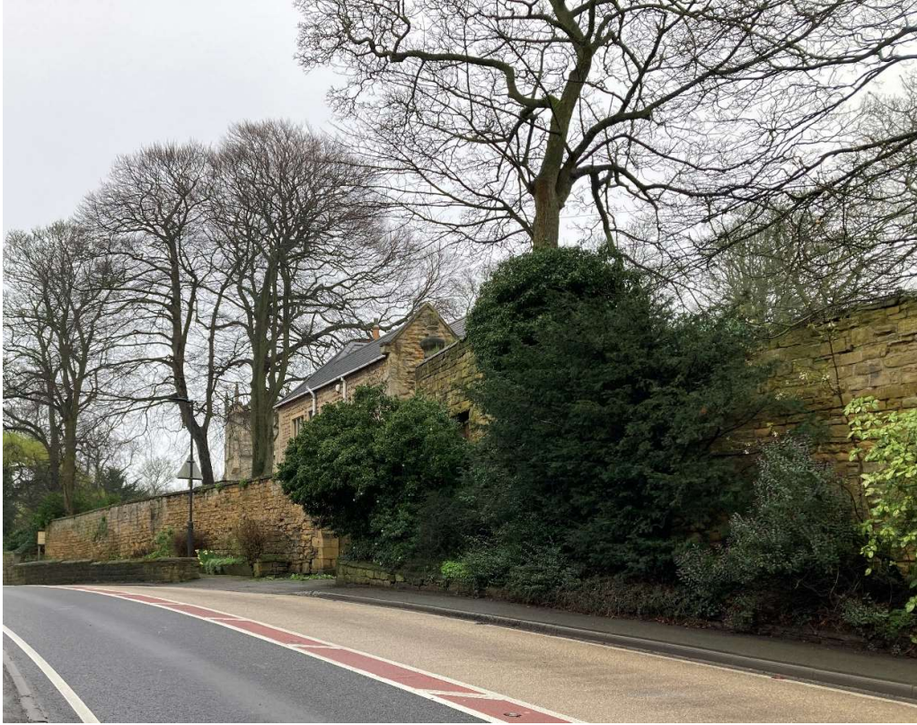
Plate 4 - Large areas of vegetation on the listed wall
