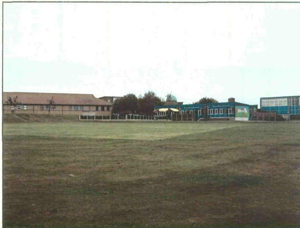
Plate 14 – St. Dominic's, looking north-west. Note embankment at left separating playing field from St. Michael's. Made ground imported during creation of field in this area.
