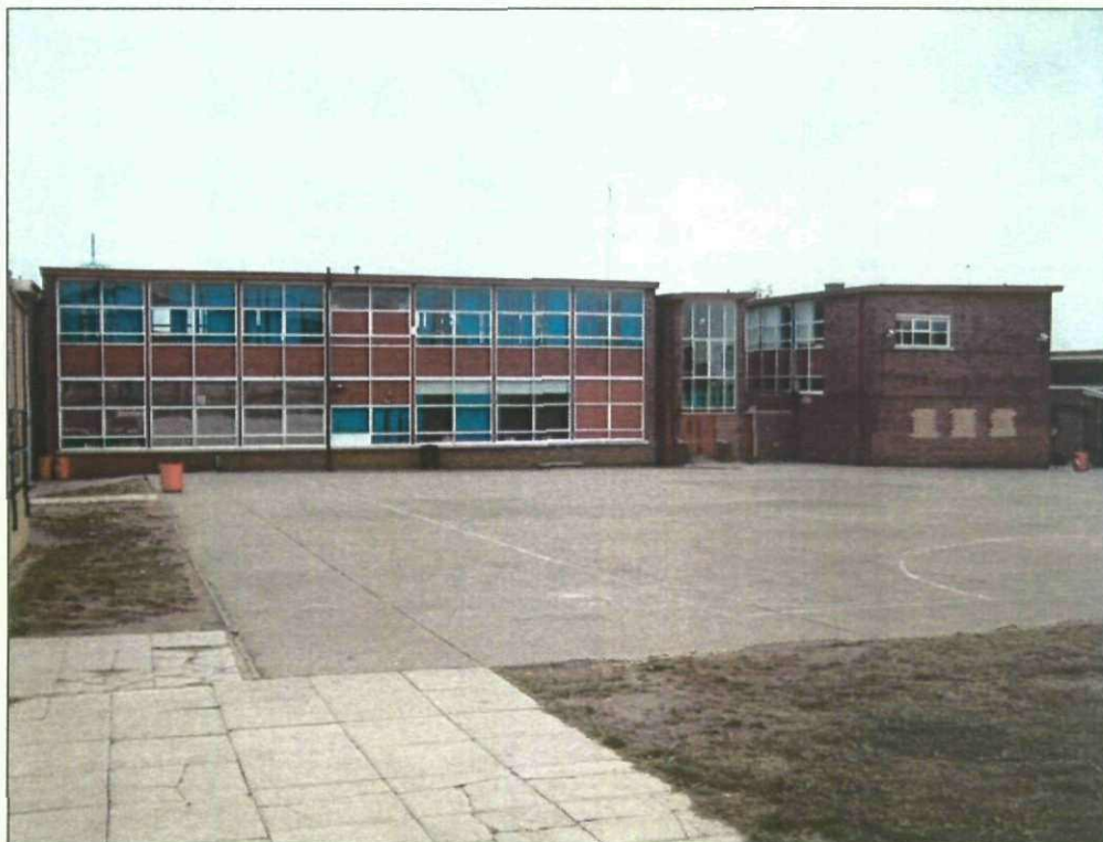
Plate 3 – 1970s block on north side of tarmac yard at St. Michael's. Part of original school construction phase.
