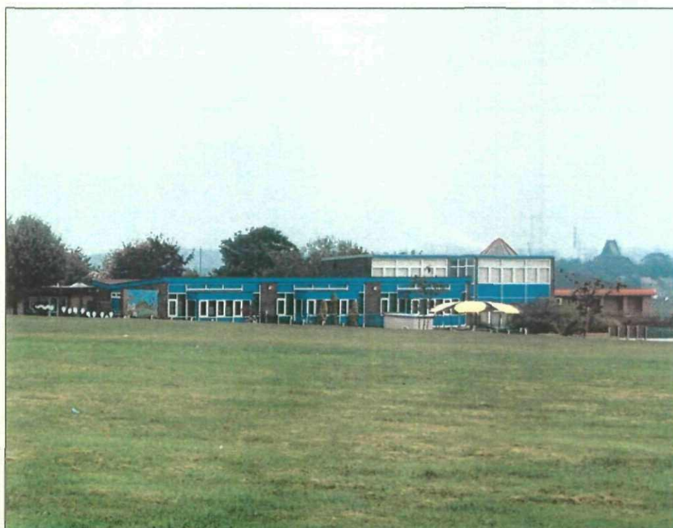
Plate 12 – St. Dominic's School, looking north-east. Made ground identified in this area by SYMAS report.
