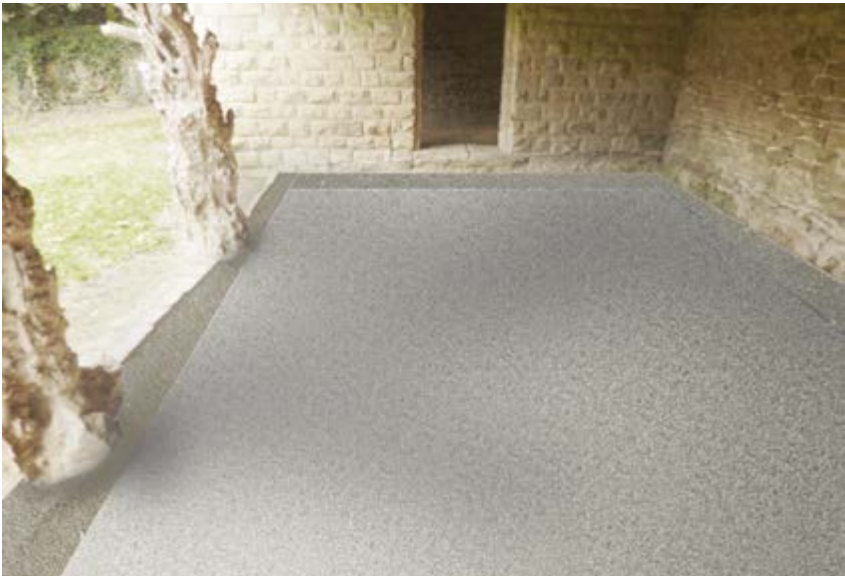
Resin Bound Gravel | Loose Gravel on the edges
