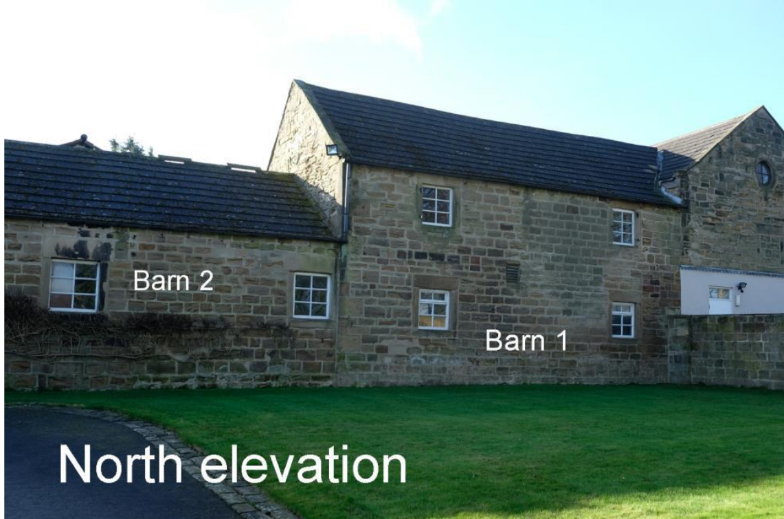
north elevation (barn 1 & 2)
