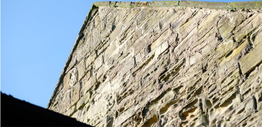
gable wall (barn 1)
