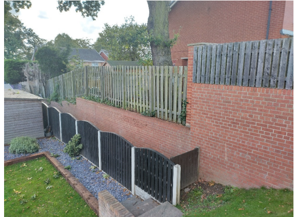
Photo 8: Retaining wall situated to east of T1, from north east
