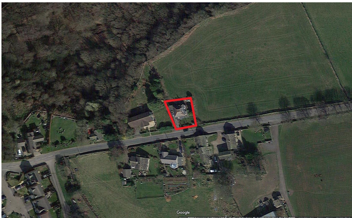
Aerial view of site
