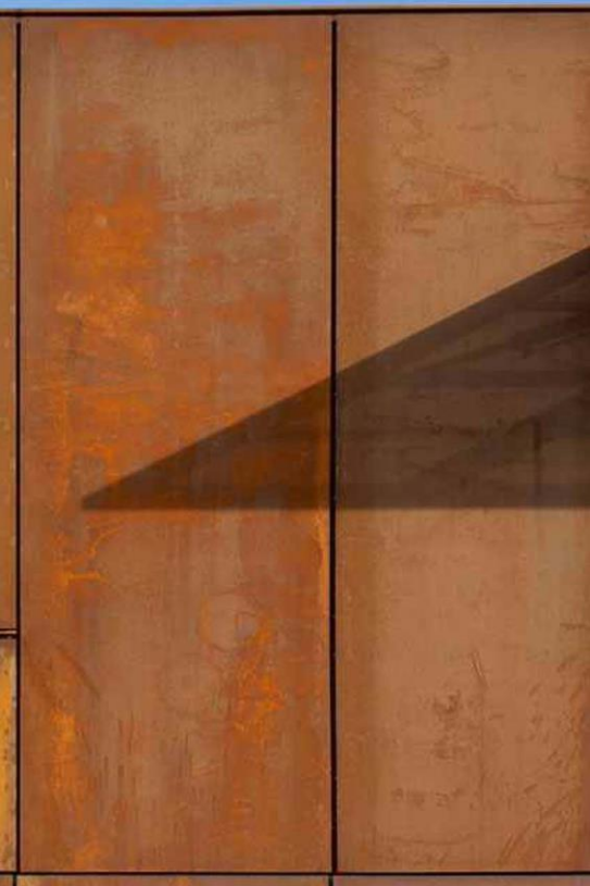
Typical corten steel panels for the walls
