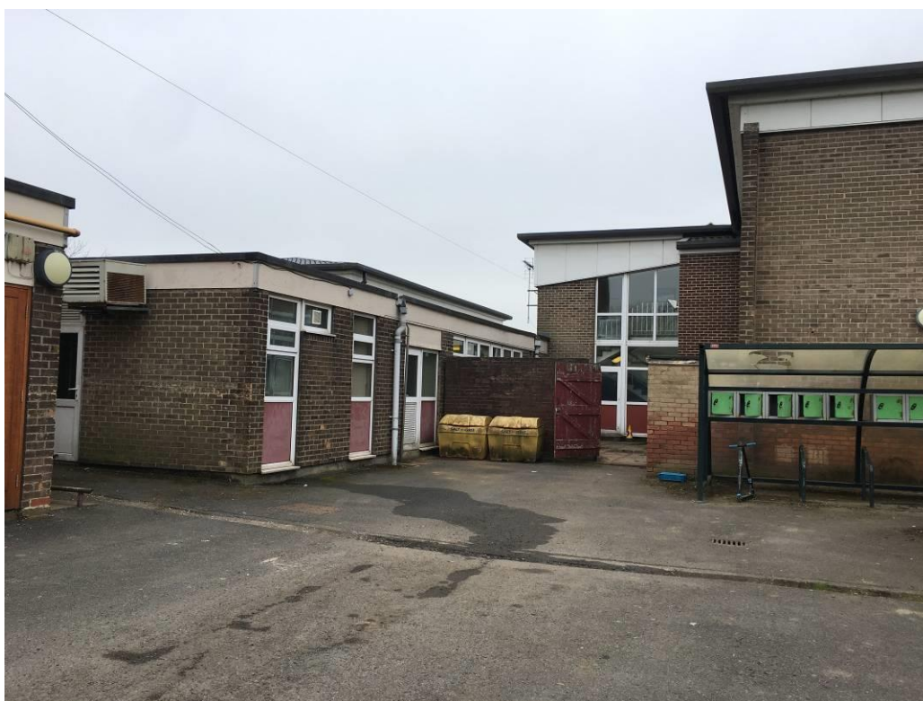
Photo 6: School buildings on site.
