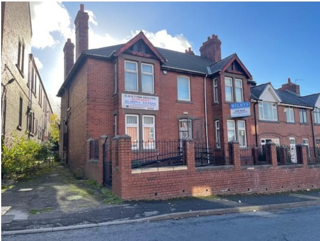
Front elevation of the building.
