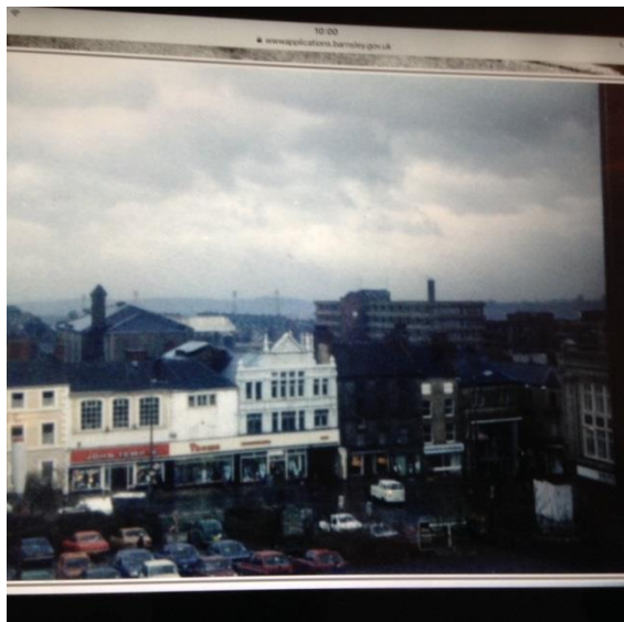
1980's view white finish to No. 16 has been removed. Old "Butterfields frontage now white.
