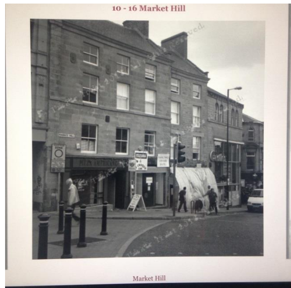
1980's picture showing a new shopfront being installed at No.16
