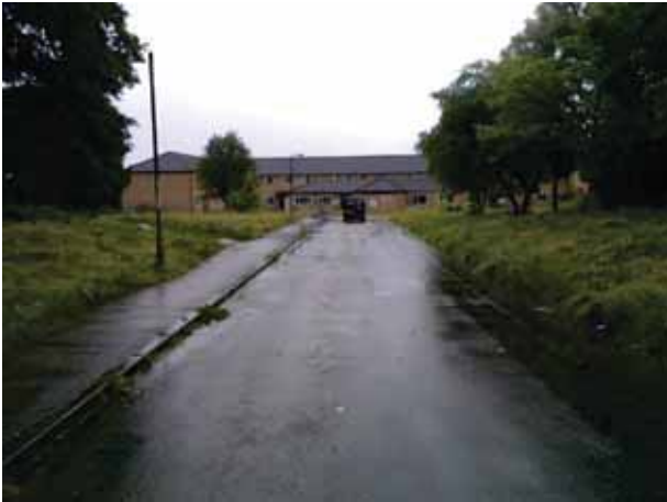
Photograph 1 (P1) View of Bolton Hall from the northern boundary (Carr Head Lane)
