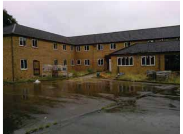
Photograph 2 (P2) View of northern side of Bolton Hall from car park to the north of the building.
