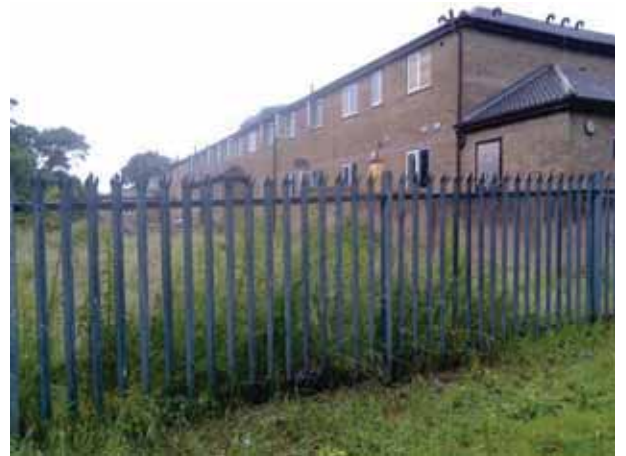
Photograph 4 (P4) View of southern side of Bolton Hall from the south east corner of the site.
