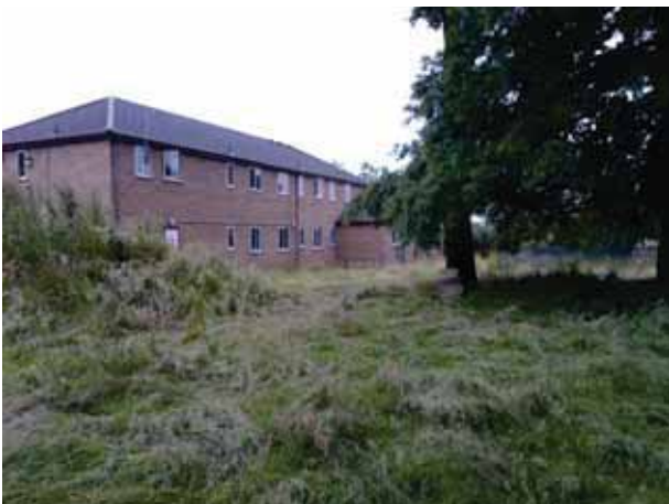
Photograph 5 (P5) View of western side of Bolton Hall from the north west corner of the site.
