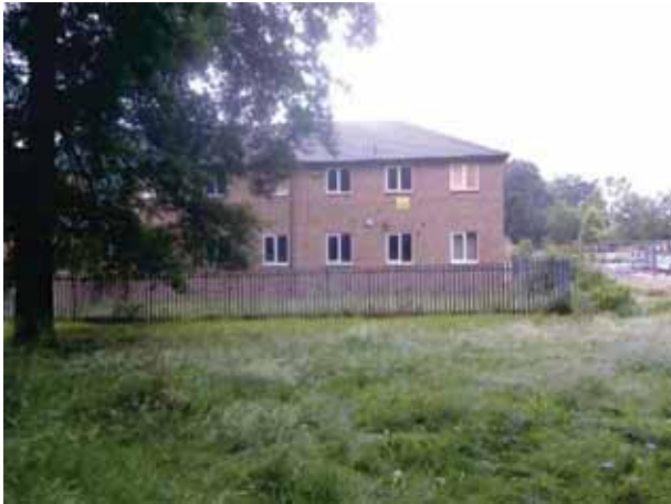
Photograph 3 (P3) View of eastern side of Bolton Hall from the eastern boundary.
