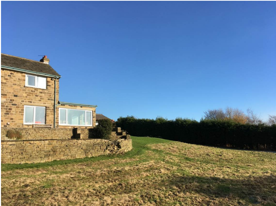
06. View of site from rear of Courtland looking east.
