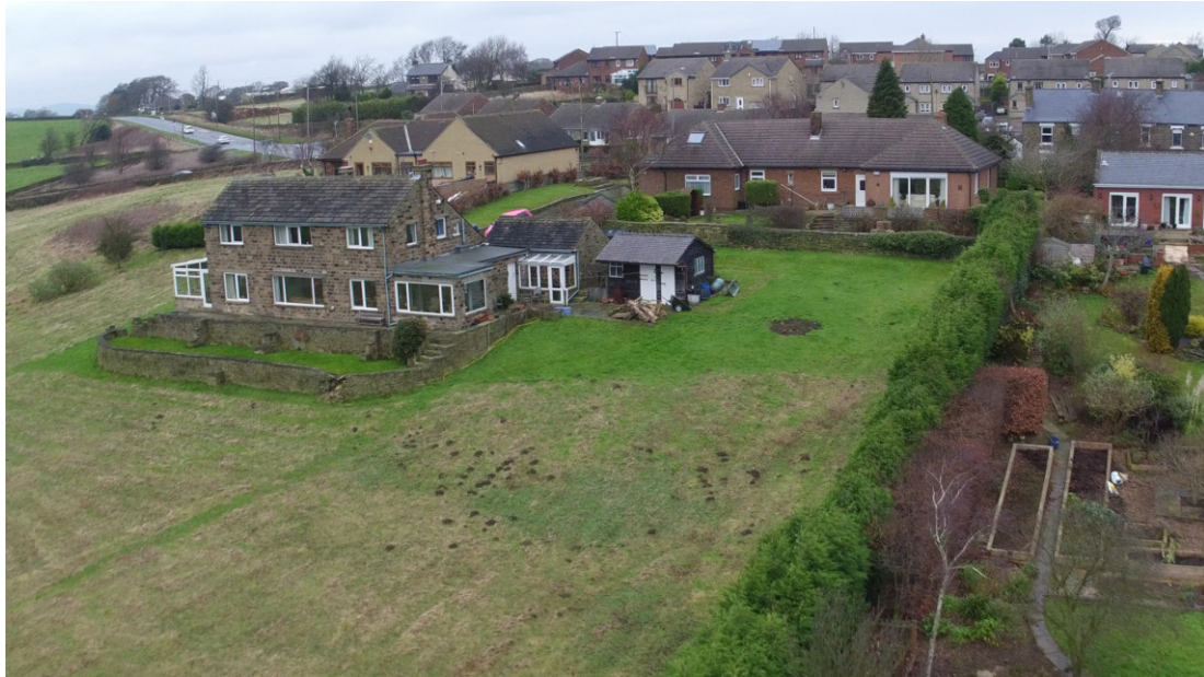
07. Aerial view taken from south east looking north west.
