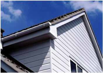
Side gables and parts of Atrium: Wood effect uPVC cladding.
