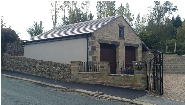
View of a similar garage in the Hoylandswaine conservation area.
