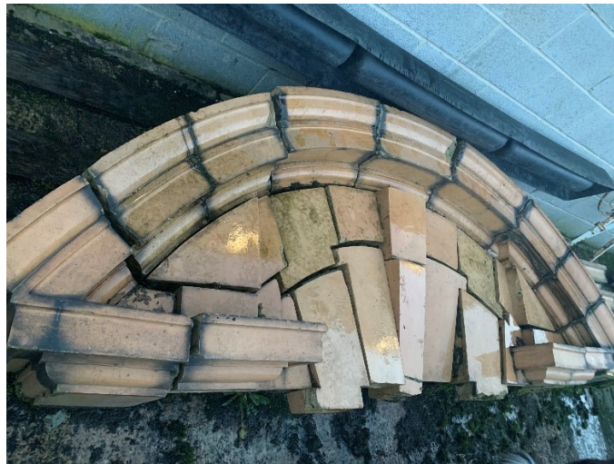
Glazed Terracotta Arch reclaimed from Miners Institute
