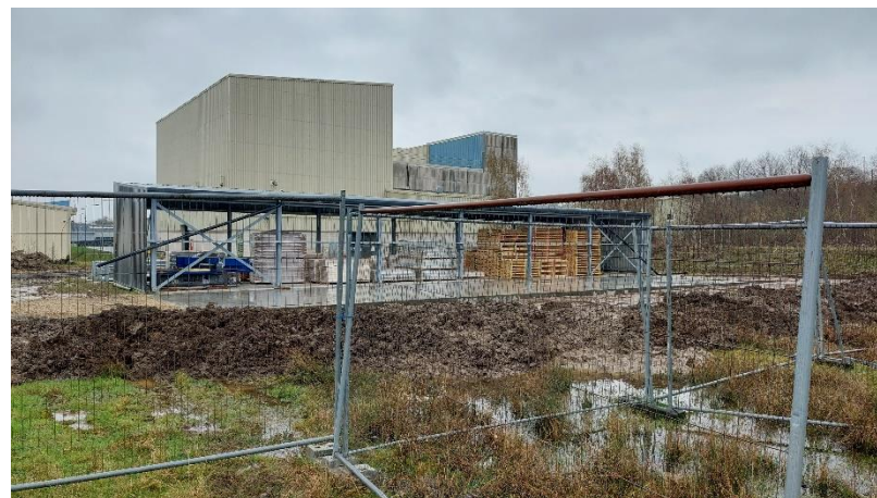
Photograph 14: Newly constructed storage area in the eastern section of the site.
