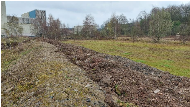
Photograph 17: Earth bund in eastern section of the site.
