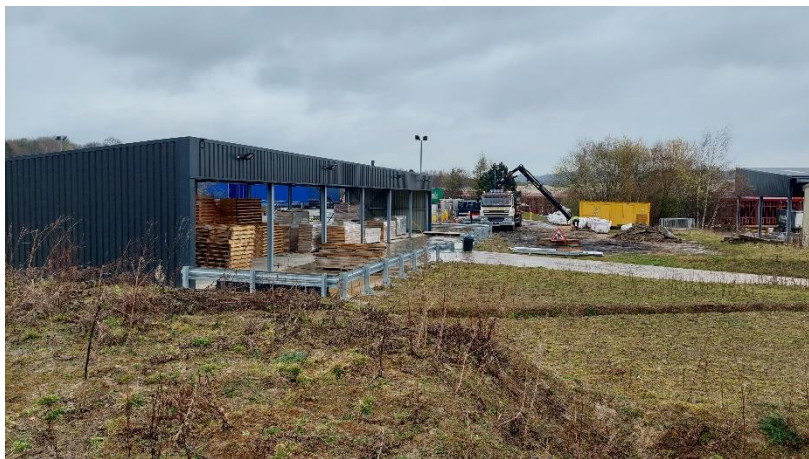
Photograph 19: Newly constructed storage area and hardstanding.
