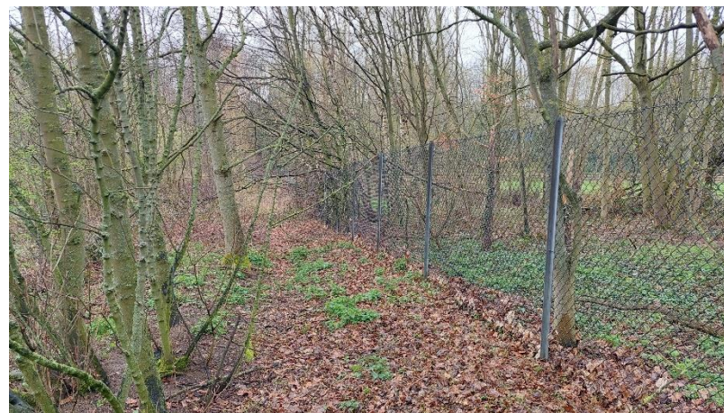
Photograph 8: Western boundary fence line.
