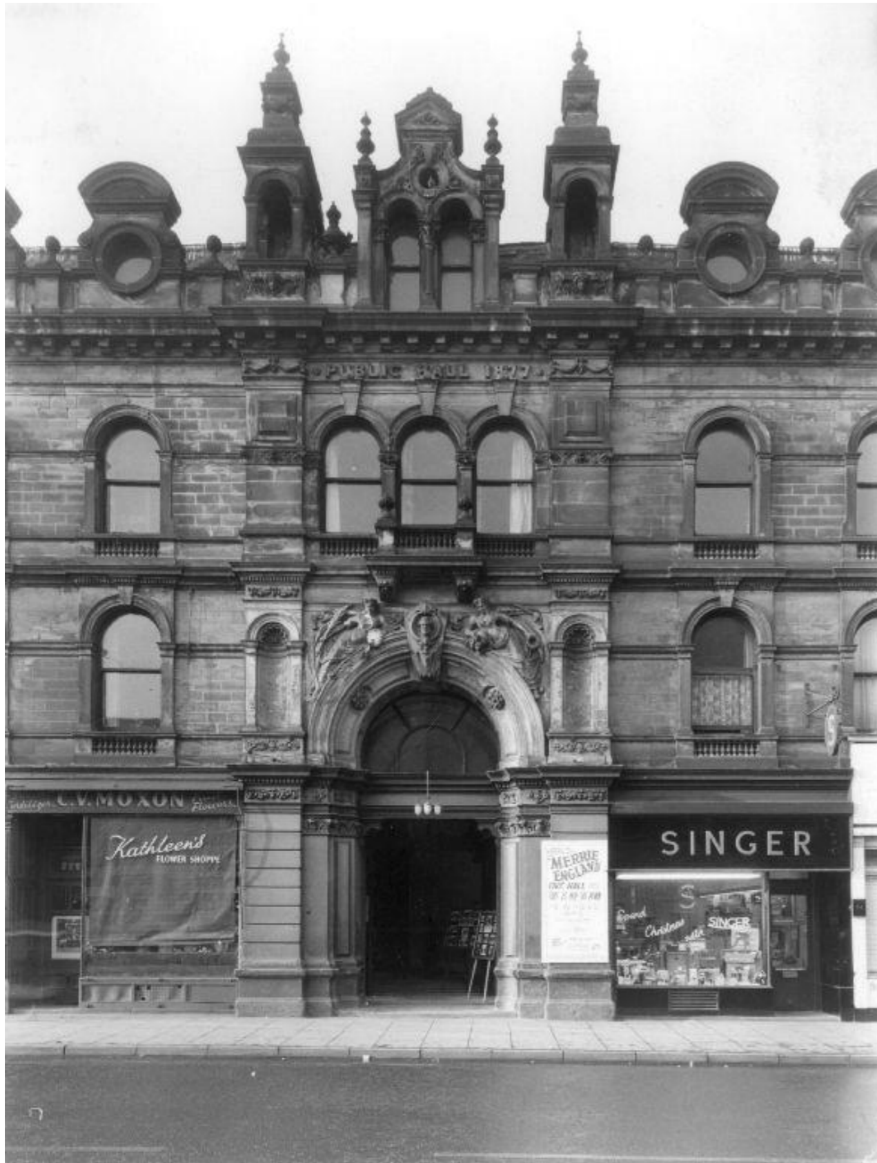
Fig. 24: Archive Image of Entrance 1963
