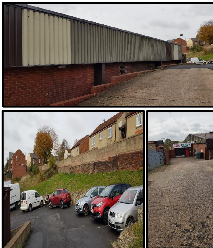
Figure 5: Hardstanding on site.
