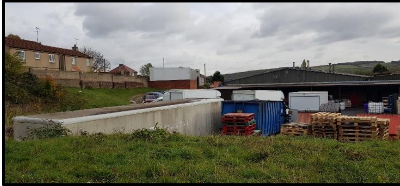
Figure 4: Storage units on site.
