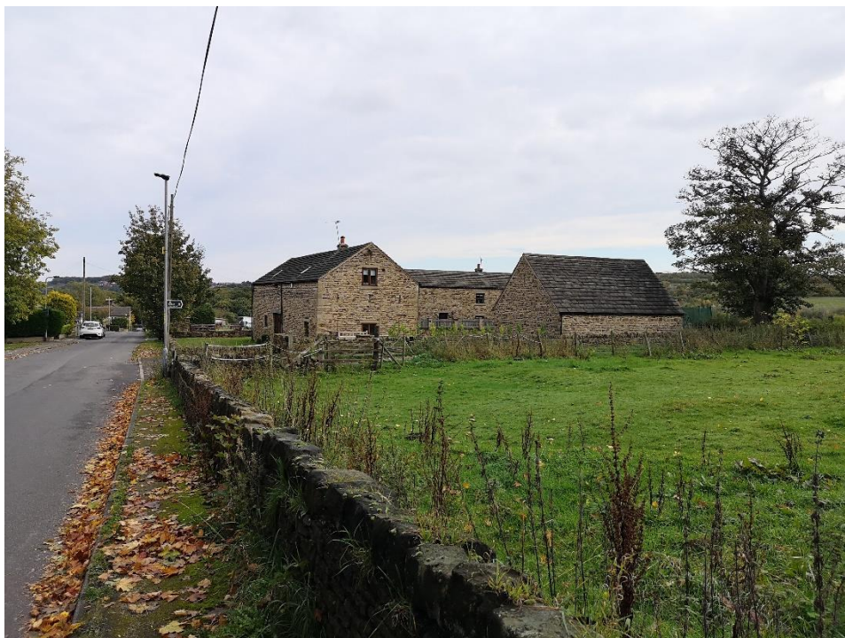
Plate 1: Listed barn NHL1315079, looking east along Hay Green Lane
