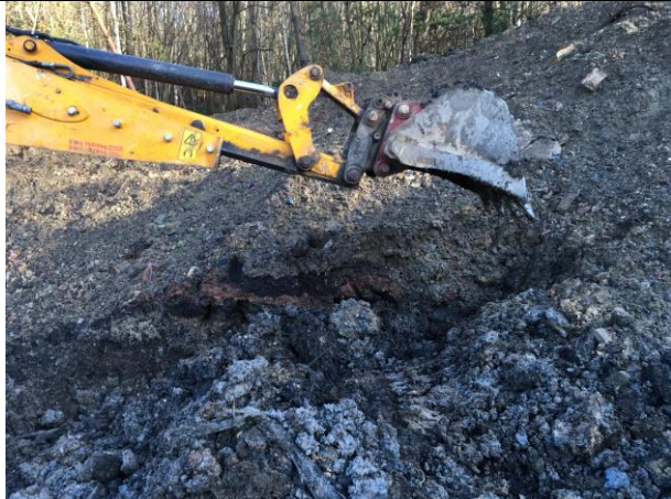
Trial pit reference STP01
