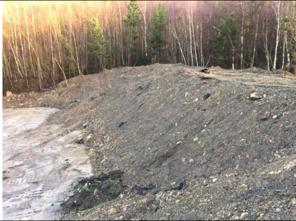
General view of stockpile, facing eastwards
