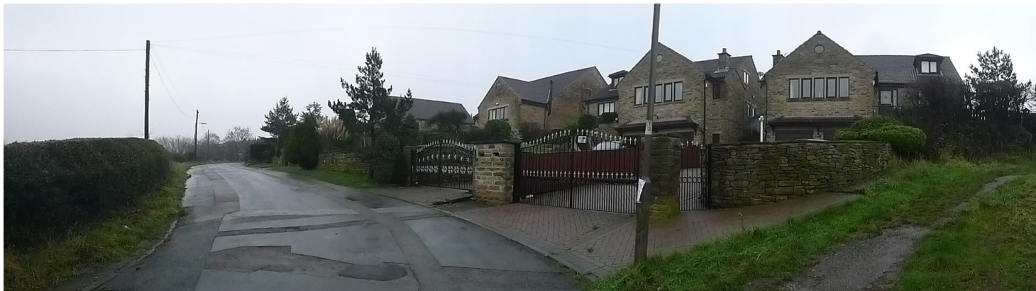
The dwellings directly adjacent to site have either stone or stone faced perimeter/retaining walls, metal gates to block paved double width driveways. The substantial dwellings appear to have been construction from approximately the 1980's period onwards, being of either stone or art.stone construction, with stone headers / cills to upvc framed glazed windows. Due to the sloping nature of their location, they have been designed with double garages at lower ground, with steps up to first floor living space along with main entrance door. The semi mature garden planting /landscaping along with surrounding lands give a semi rural identity /character to the current street scene. Which is not the case along the entire length of Upper Hoyland Road.
