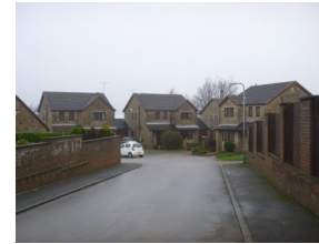
Mid size dwellings of Art. stone, recently constructed, access road perimeter wall is constructed with red brick pier and timber fencing infill panels.
