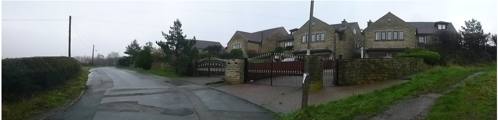
Existing dwellings with double garages overlooking proposed site.
