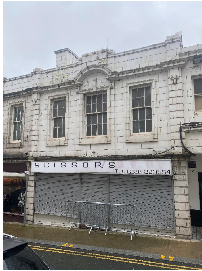
1.3 Current redundant shop unit with security shutters and Function Room over
