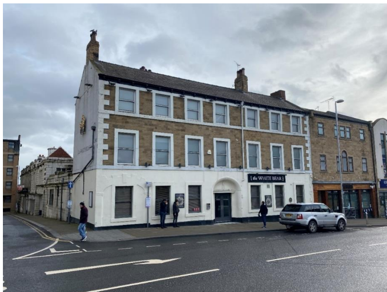
1.0 Front façade from Church Street
