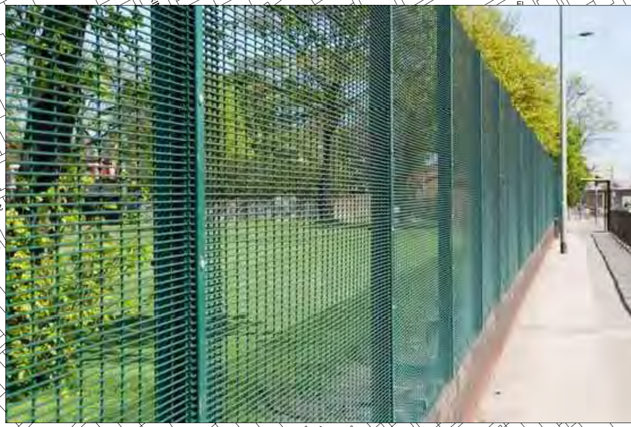
2.4m high Paladin (weldmesh) Fencing Dark Green RAL.6005, to boundary
