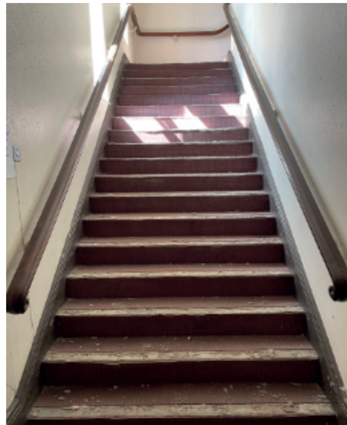
Former public staircase to Court Rooms
