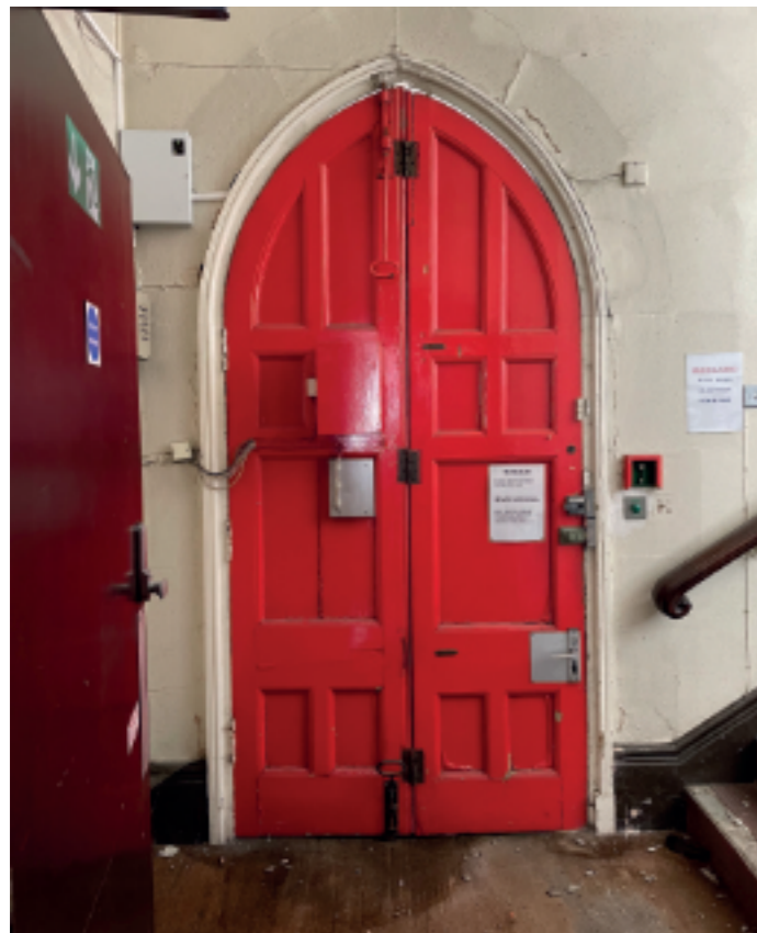
Westgate Main Entrance interior
