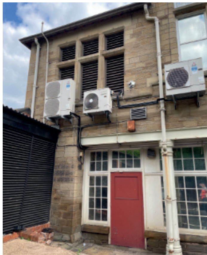
Western entrances (northern door/fire escape)
