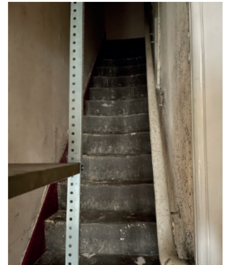
Prisoner's stair interior (blocked to First Floor)
