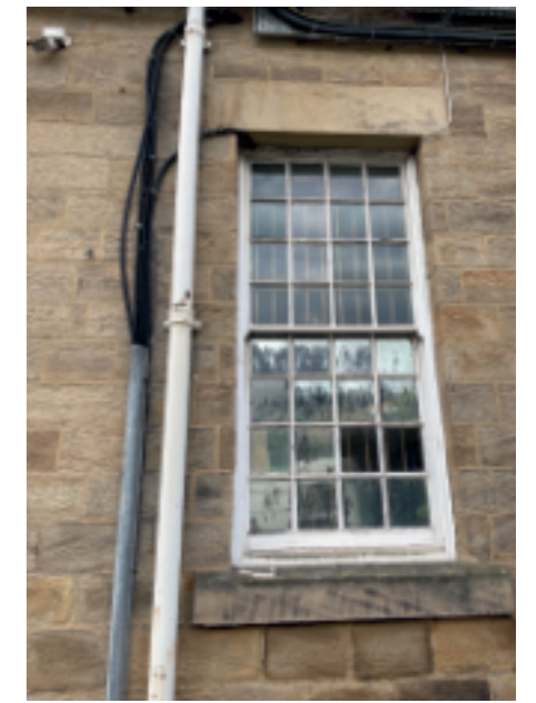
Northern façade window
