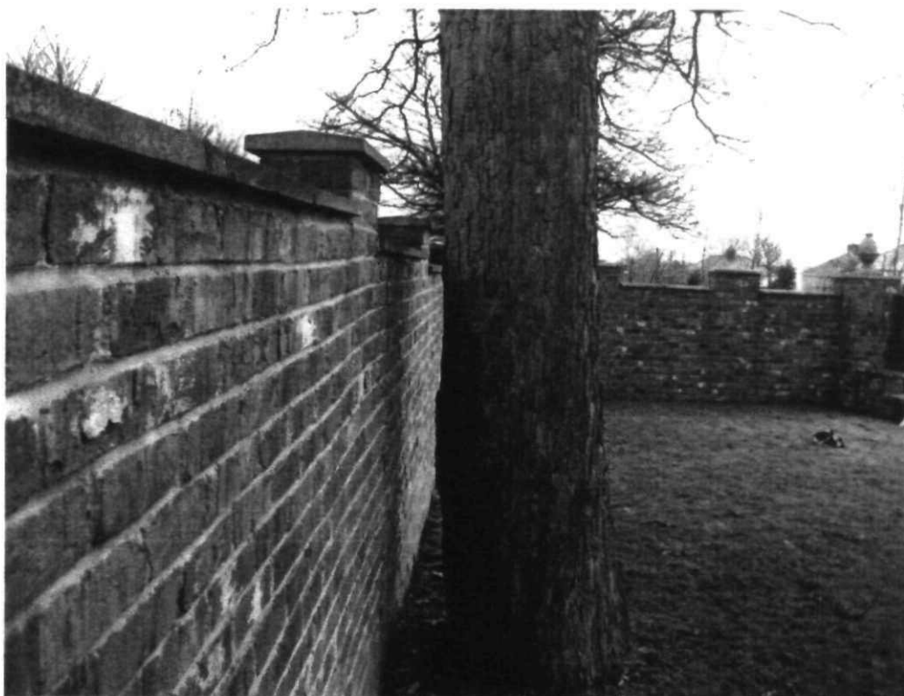
Photograph 5 shows stem of sycamore tree T4 in relation to the existing 2000mm high boundary wall.
