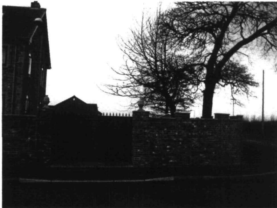
Photograph 2 showing the gated entry off George Street adjacent to the junction with Middlecliffe Lane. Photograph also indicates the 2.000metre high perimeter brickwork wall which forms the boundary of the site.
