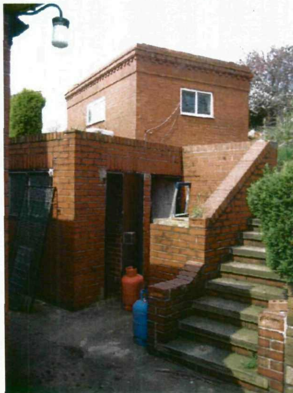
6. Access steps and retaining walls illustrating a change in level between the detached garage and existing bungalow.
