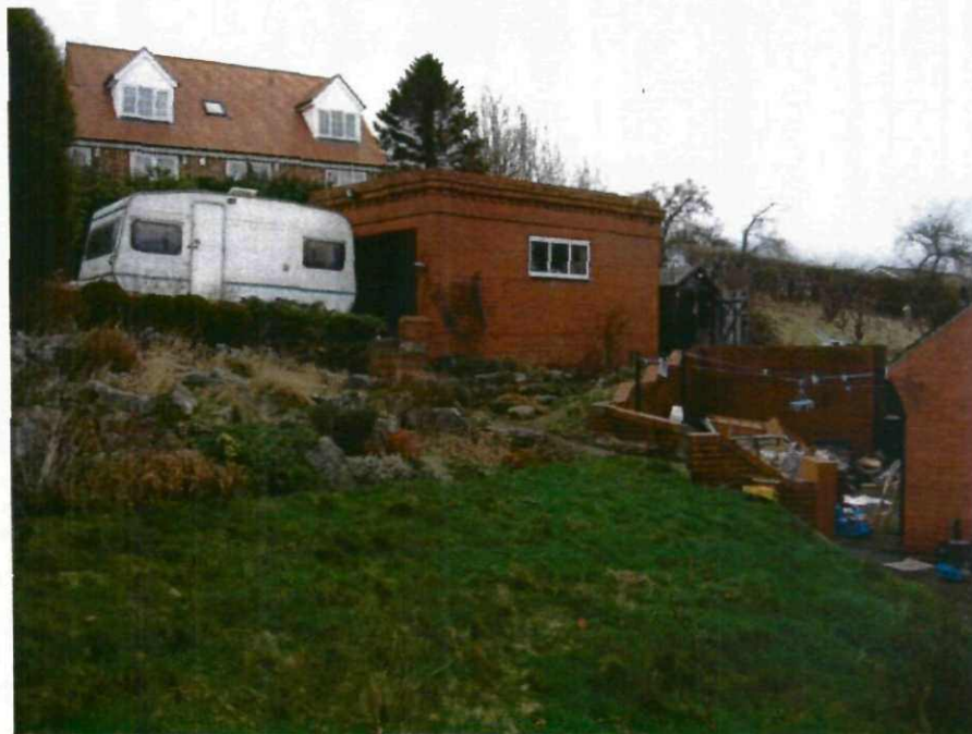
4. Existing detached flat roofed garage at the upper level.
