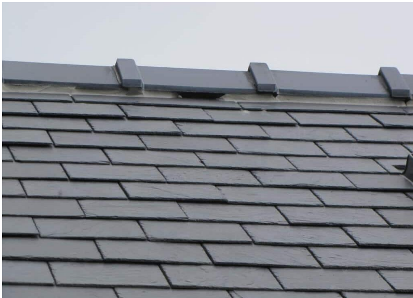
Figure 4. Example if bat access point in the ridge
