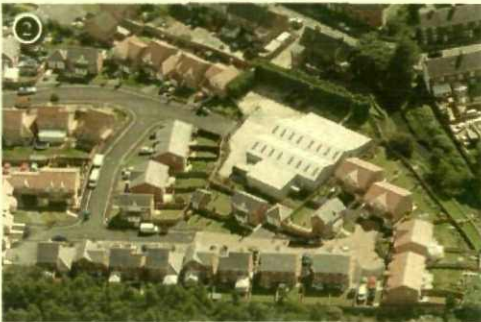
More recent residential development to the north east of the site are semi detached in form and predominantly 2 storeys in height.
