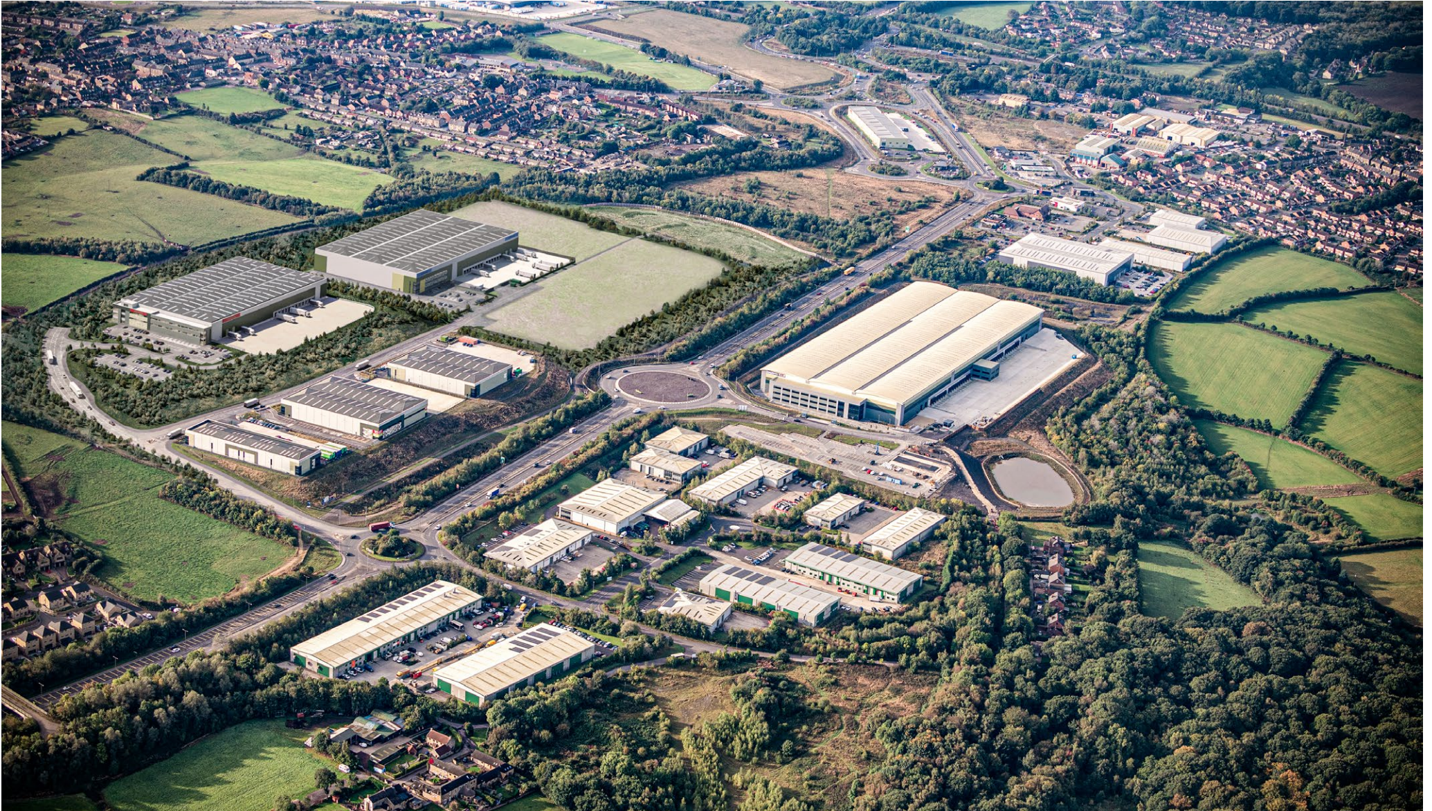
Aerial CGI of Phase 2B - In response to Condition 25(c) - 3D Aerial View
