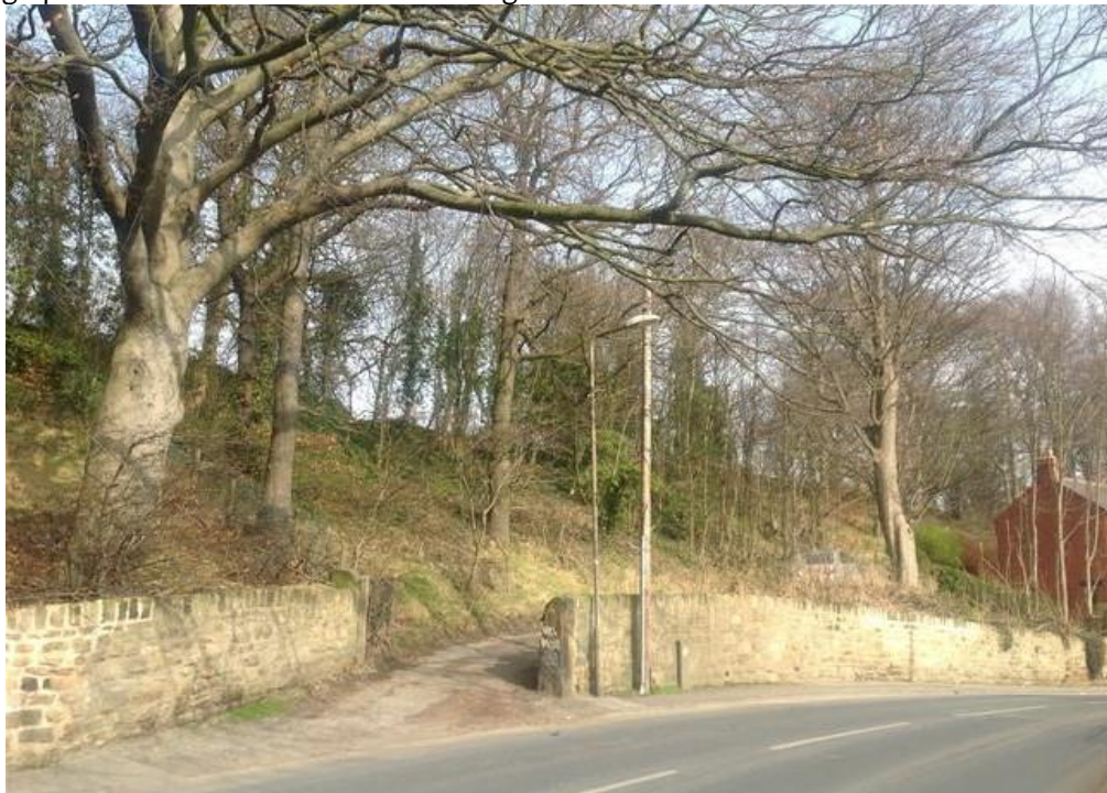
Photograph 2. Track entrance viewed from Kingwell Road.
