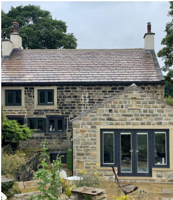
Fig 01. White House Farm new stone roof.
