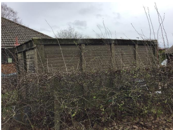
General view of the rear elevation of the garage
