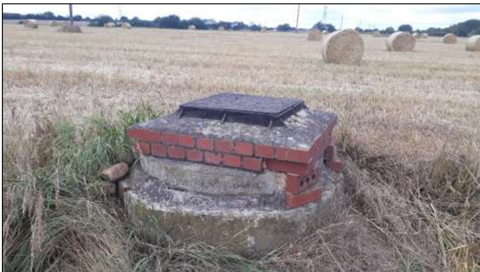
Plate 6: Inspection shaft to underground utility aligned parallel to OHL
