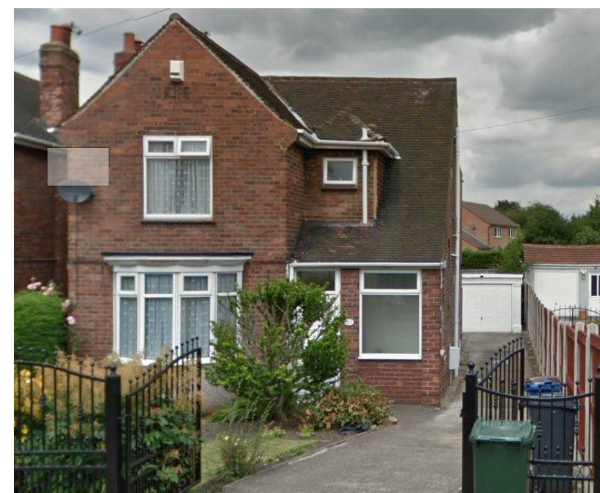
EXISTING FRONT VIEW SHOWING DRIVE AND EXISTING GARAGE FRONT
