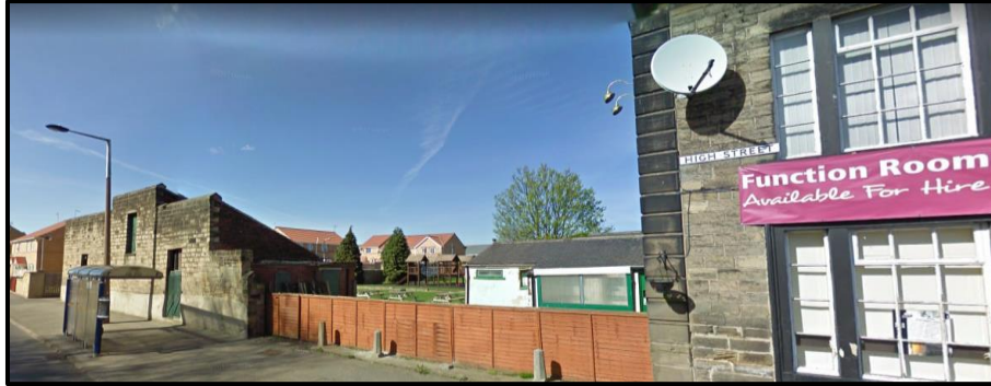
Photograph 3 – View of the site from High Street
