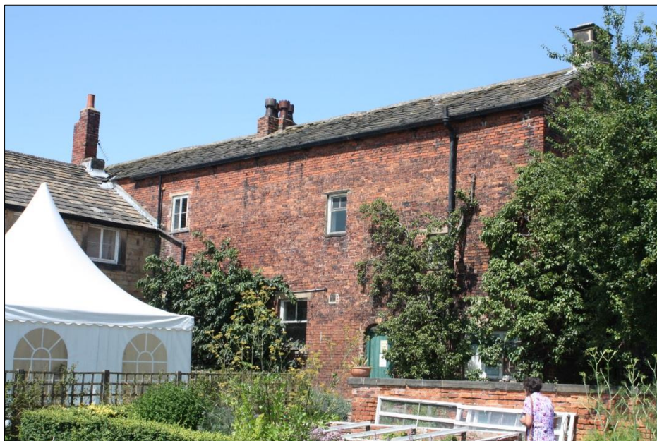
COTTAGE NO 2 – REAR ELEVATION FACING SOUTH
