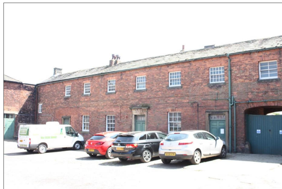
COTTAGE NO 2 – FRONT ELEVATION TO STABLE YARD
