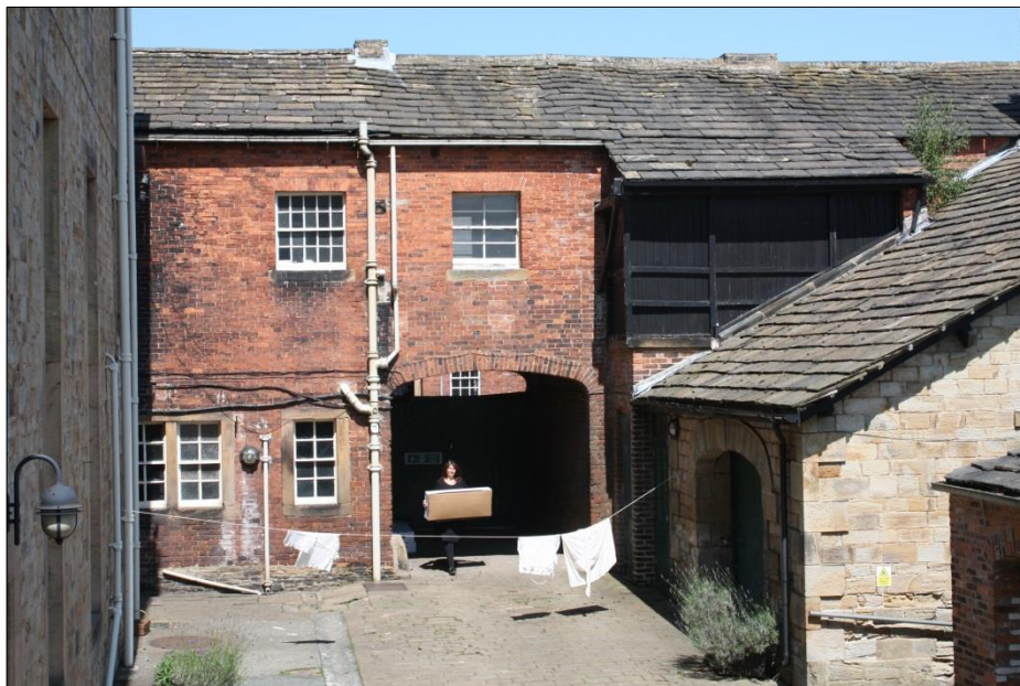
COTTAGE NO 1 – REAR ELEVATION FACING SOUTH
