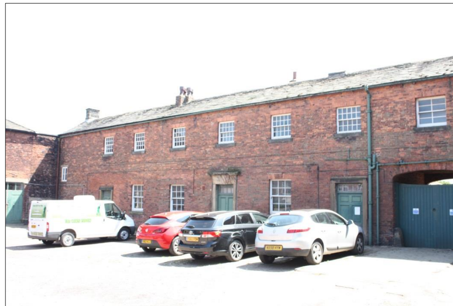
COTTAGE NO 1 – FRONT ELEVATION TO STABLE YARD
